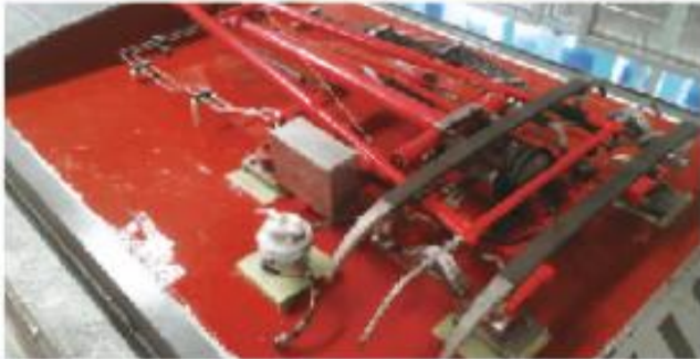
Flat top scraping and roller coating construction;
