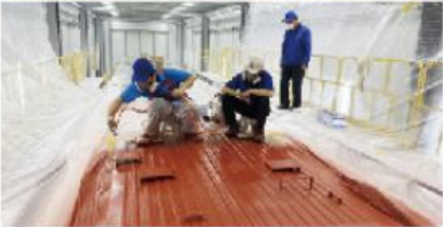
Corrugated roof spraying construction
